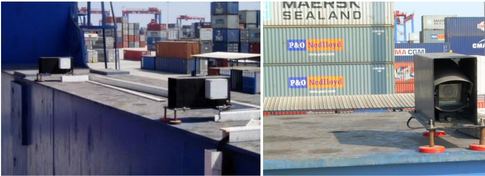
STS crane mounted Cameras on sill beam
